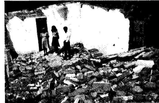
The adobe home of the Arreagas of Guatemala City could not withstand the earthquake.
