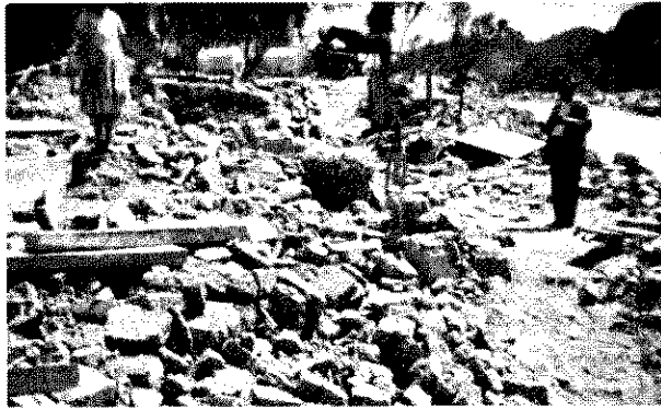
The remains of the church at Zaragoza, one of 13 churches which were completely destroyed.
